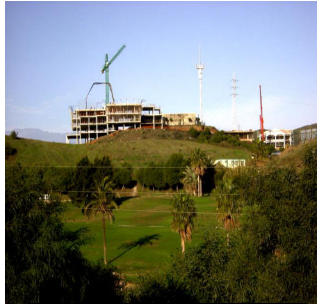
Altos Phase 2, Structure Build. VII, Dec 2000
